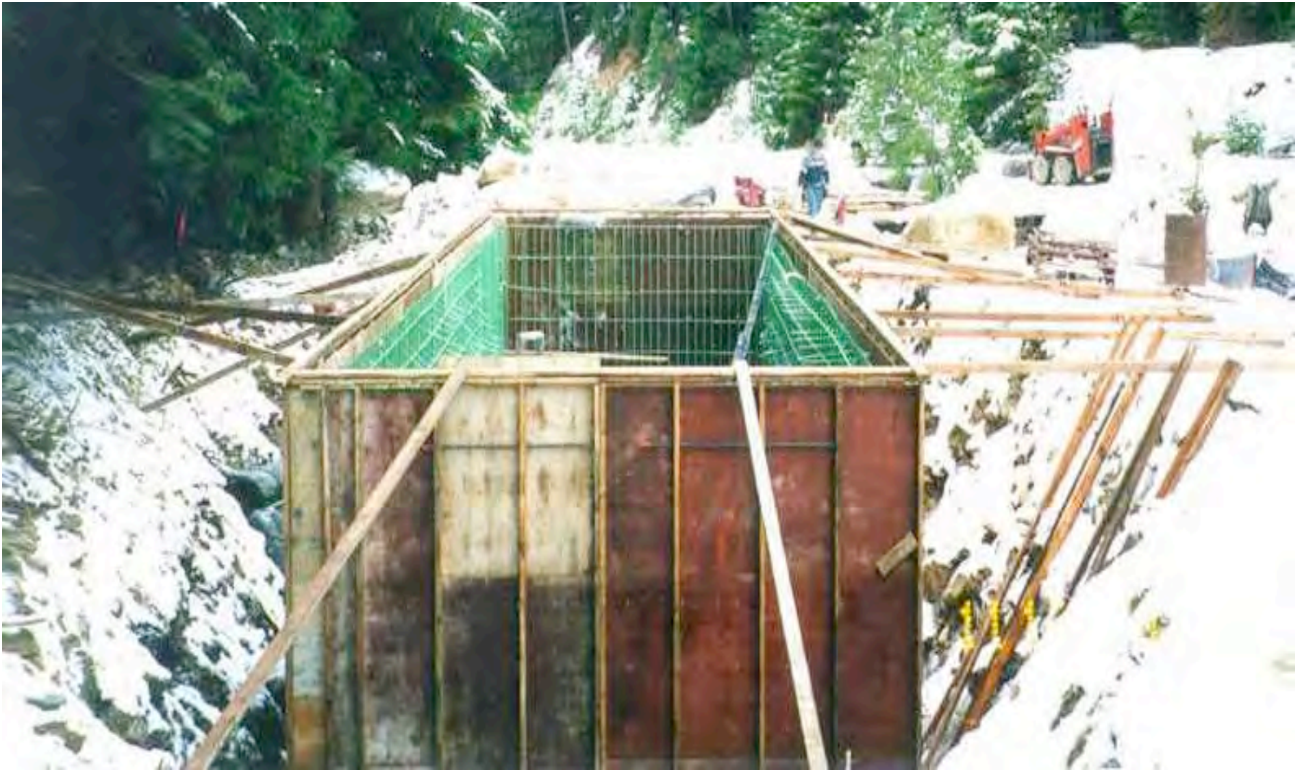
Construction of PRB vault between East Fork of Ninemile Creek and the Tailings Pile.
